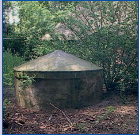
the well before restoration
